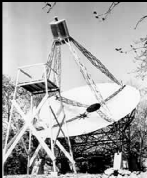
Reber's Radio Telescope, 1937
