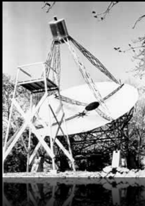
Reber's Radio Telescope, 1937
