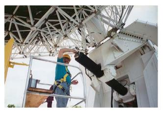
Figure 1: Left, the SMA antenna mount, made of 130 mm thick steel plate to meet the antenna stiffness requirements for pointing. Above, detail of the interface between the antenna pedestal and the reflector assembly. Note the ball-screw drive and the four flex-pivots used to connect the carbon fiber central hub of the reflector assembly to the steel weldment that connects to the elevation axis and screw drive.
