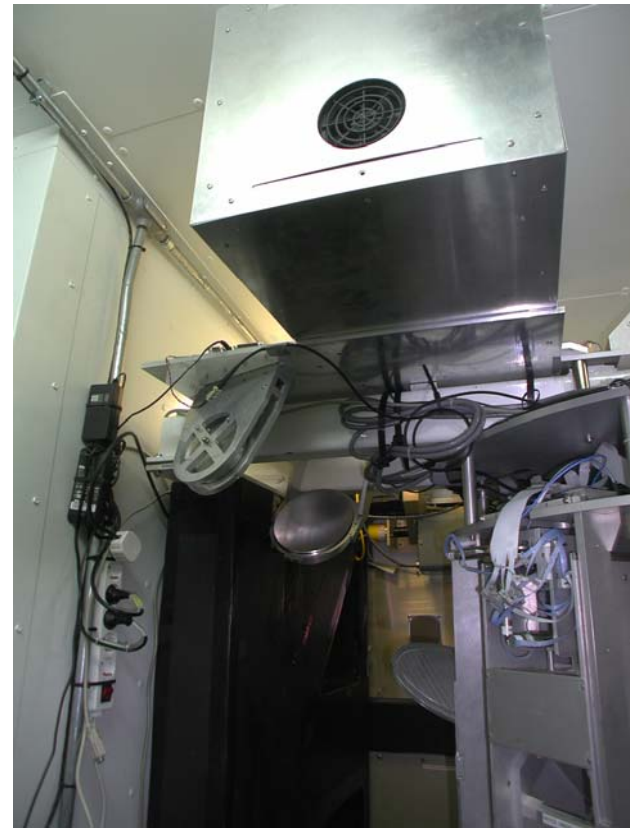
WVRs installed into Antennas 5 and 6
