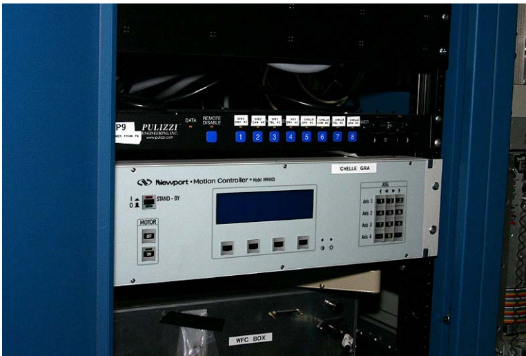
Figure 58. Pulizzi 9 and the Hectochelle grating controller.
