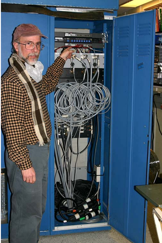
Figure 55. Dome calibration control. To operate the dome calibration lamps make sure that the green-coded power connector on the bottom of the rack is connected and that the Pulizzi at the top of the rack is on.
